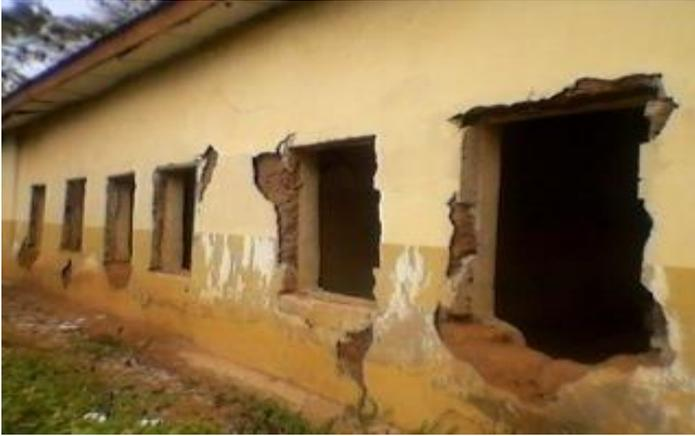
Fig. 3. Damaged classroom windows, not repaired but still in use.
